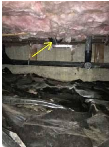
Photo 15-2 Leaking p-trap.
