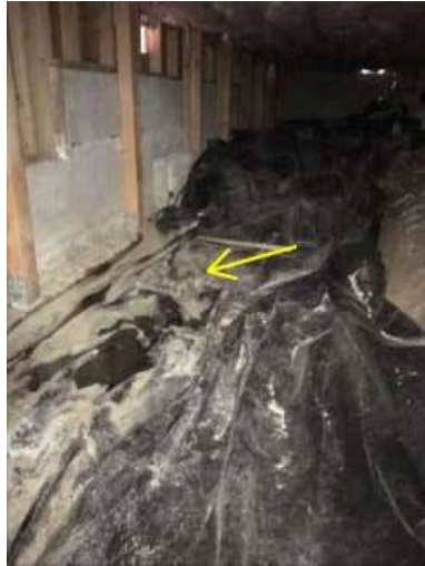
Photo 18-4 The light/white coloring on top is sediment staining.
