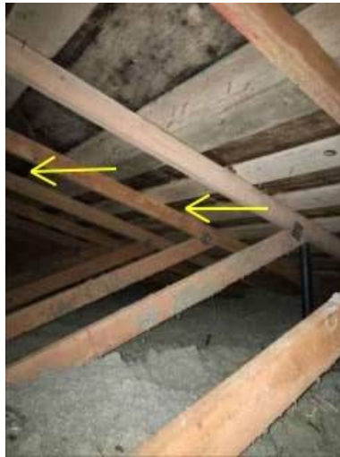
Photo 10-2 White growth, such as that observed here, during the inspection, can be mitigated by removing the source of excessive moisture. Once the moisture is eliminated the microorganism can no longer grow.
