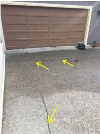
Photo X-15 Driveway cracking.
